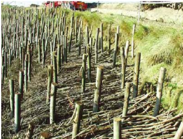
Once brushwood mattress installation is complete, rock netting is secured to the posts to prevent wash out – 2005
