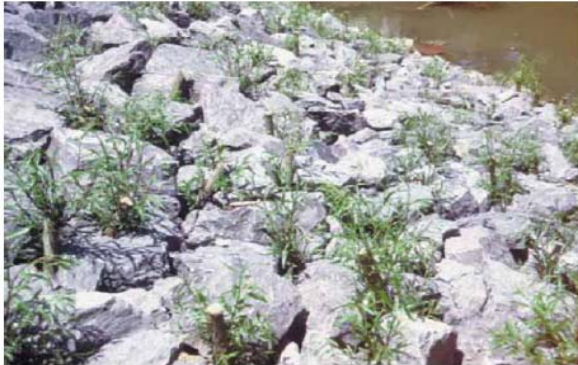
Vegetated Riprap along Stream Bank
