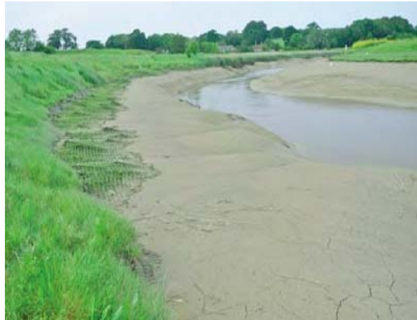
Seven years post-restoration the structure has continued to retain sediments and has been stabilised further by vegetation
