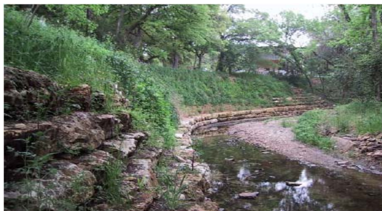
VEGETATED MECHANICALLY STABILIZED EARTH (MSE) WALLS
